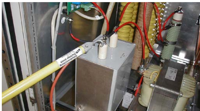
Single-pole device for discharging static charges.
