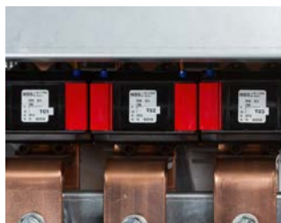
Built-in protective current transformers
