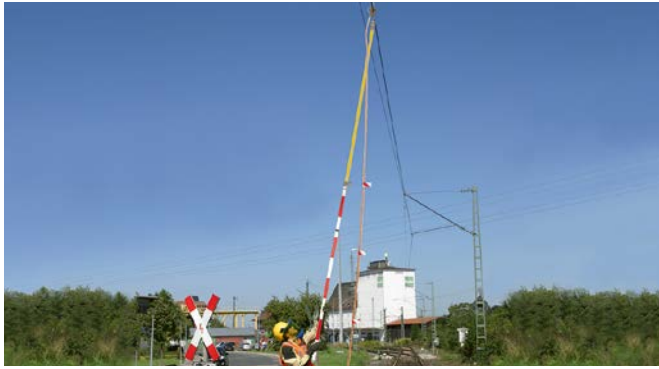
Attaching a railway earthing device.
