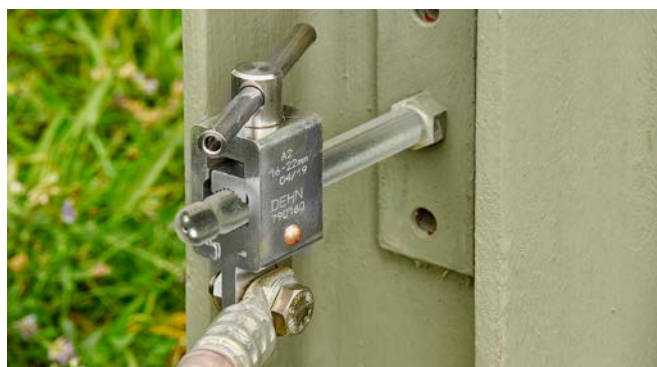
Earth bushing with tommy bar on a fixed earthing point with ring groove.
