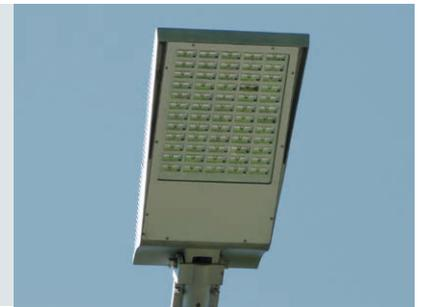
LED mast lights for street, walkway and open space lighting are mounted at light point heights of several metres to ensure a large field of illumination. This, however, is only possible if the luminous flux of the light source is sufficiently high which is no problem for today's highly efficient LEDs. Their long service life, almost independent temperature sensitivity and individual setting of different scenes make them cost-effective and environmentally-friendly.
