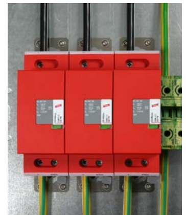
The arrester can be mounted on a mounting plate using the two mounting brackets provided.
